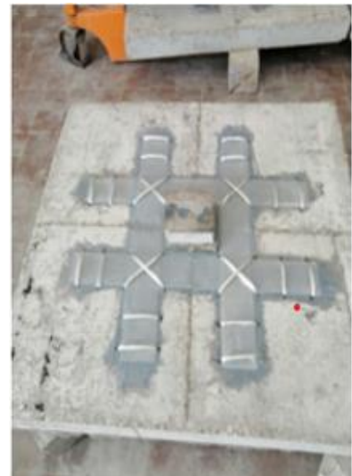
fixed the studs on their places
