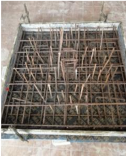
location of holes before casting
