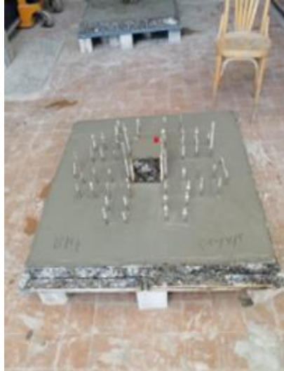
just after casting concrete
