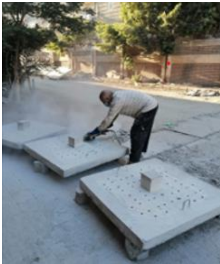
levelling the bottom surface of the slab by using grinder
